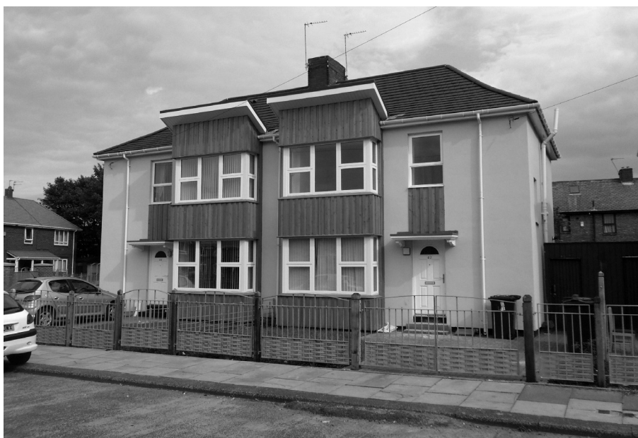
Figure 4. Systems in situ: both bays in place, after minimal disruption
