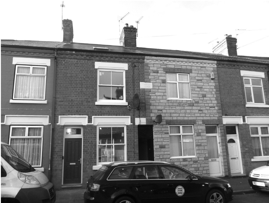
Figure 2. snug fit: the completed property, with an additional room in the roof to compensate for the loss of internal space
